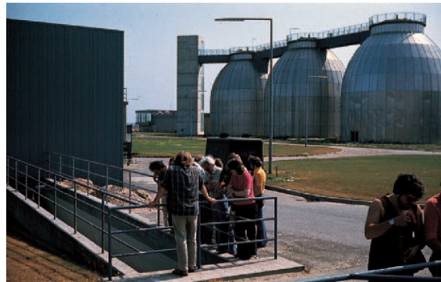
Figure 29.28 High-Efficiency Anaerobic Bioreactors Used for Sludge Digestion and Methane Production. These “egg-shaped” units are so well insulated that they maintain their temperature (39°C) without outside heating, and the methane can be burned to provide electricity. These reactors are located at Kiel, Germany.
